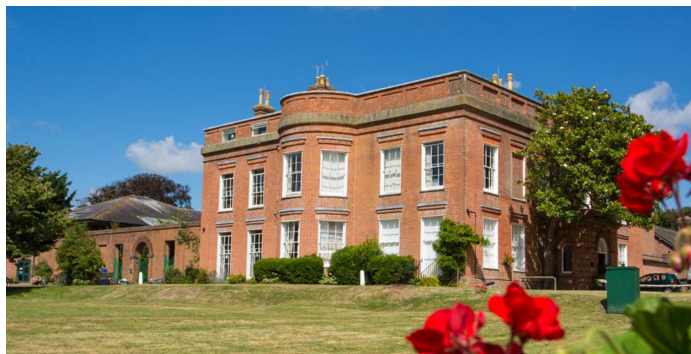
Grade II Listed Goring Hall
